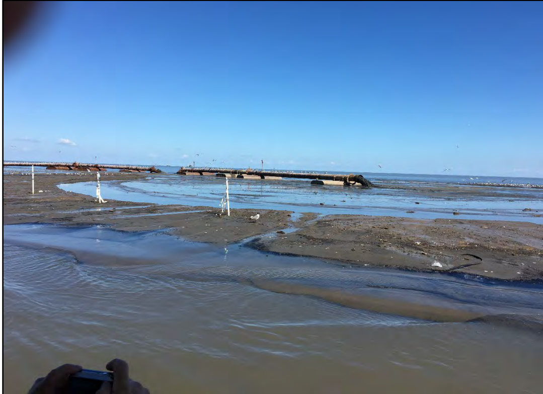
23 June 2016: Gunn Island with on-going dredge discharge
