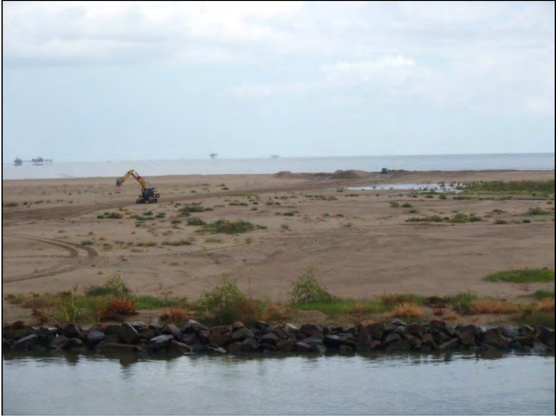
7 October 2011: Marsh Creation Site G (Contract 11-C-0015) looking east over jetties
